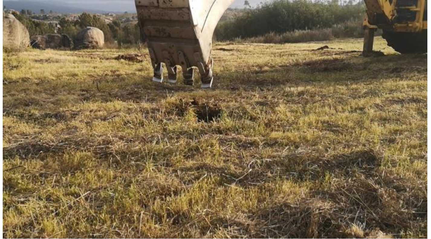
using a backhoe
