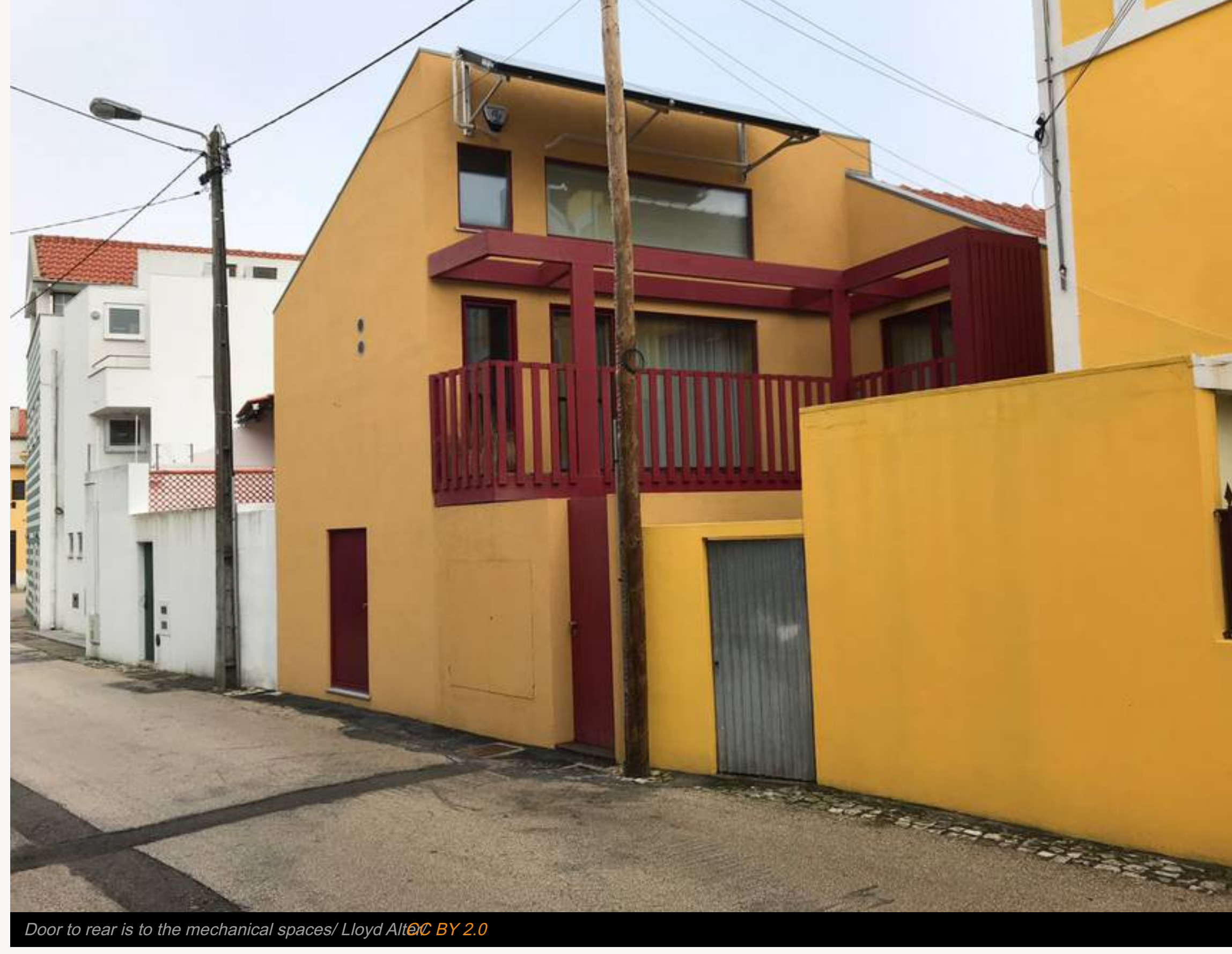
Door to rear is to the mechanical spaces/ Lloyd Alter/CC BY 2.0
